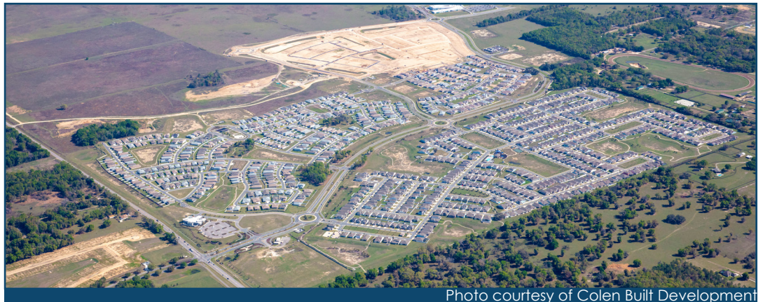
Aerial view of Calesa Township.
