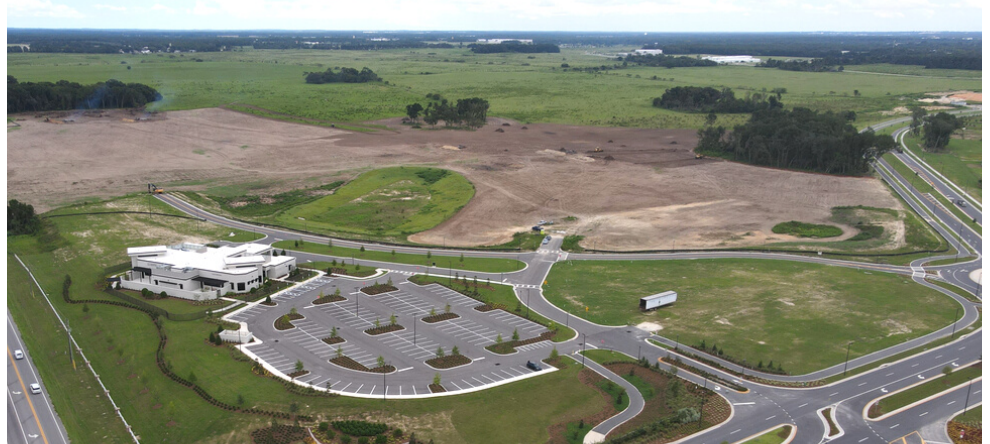
Land development progresses in the next neighborhood of Sorrel Glen.
