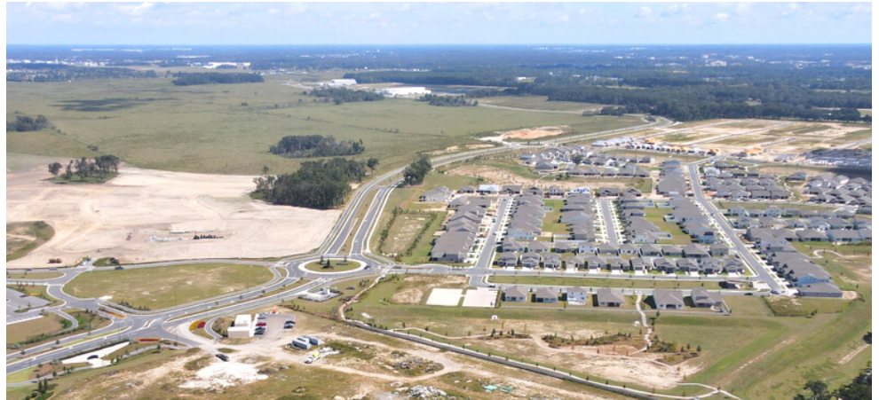
Progress continues in the second phase of Roan Hills and Sorrel Glen.
